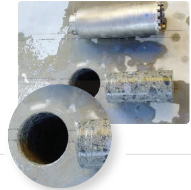
2- We remove the center pin when the CORE BIT has penetrated slightly.
